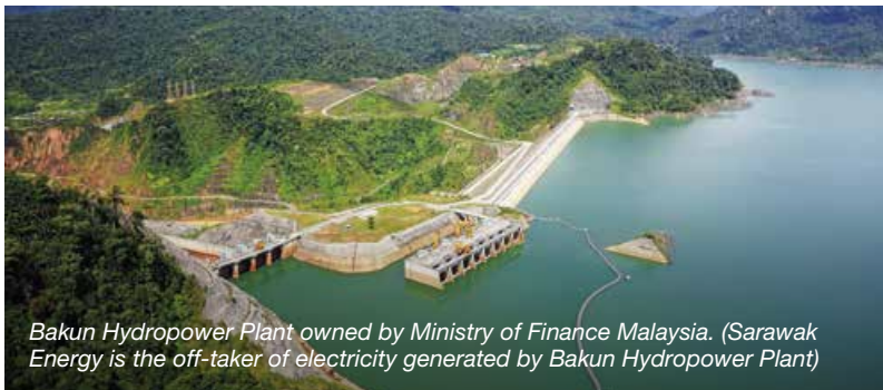
Ecological Power Plant
