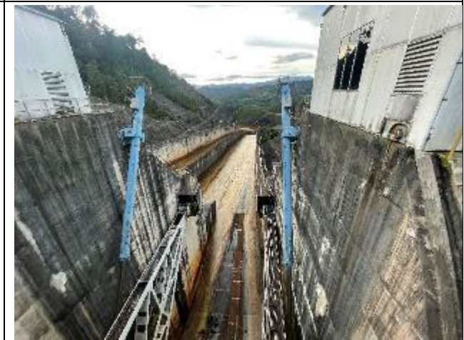
Photo 66: Spillway radial gate
