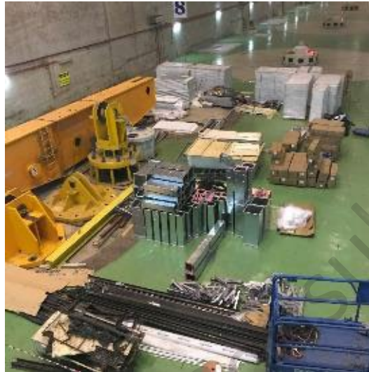
Photo 20: Tidy storage of equipment and materials during works, turbine hall
