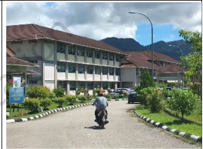
Photo 75: Sungai Asap secondary school
