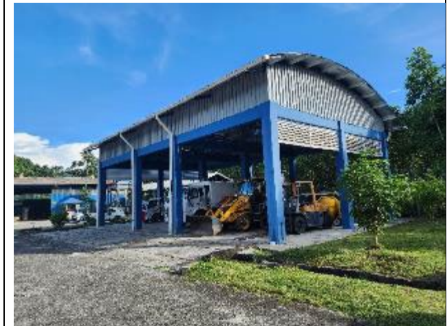
Photo 24: Covered areas for major equipment at Bakun HEP
