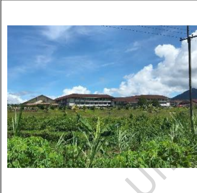
Photo 76: Sungai Asap secondary school
