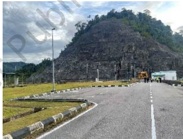
Photo 71: Bakun left abutment
